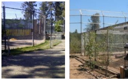
Compliant big cat fencing
